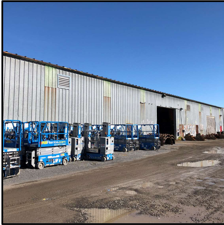
Photograph 1: View of subject building looking north.
