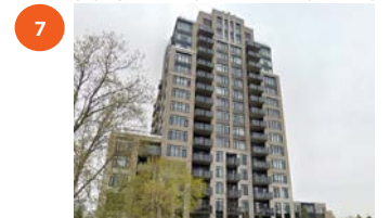
75 CLEARY AVE. 16-STORY RESIDENTIAL BUILDING
