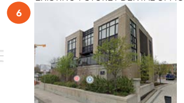
773 RICHMOND RD. 3-STORY RESIDENTIAL BUILDING
