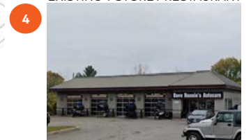
801 RICHMOND RD. EXISTING 1-STORY AUTO SHOP
