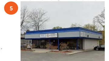
797 RICHMOND RD. EXISTING 1-STORY DENTAL OFFICE
