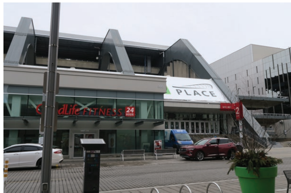
Western portion of the podium on the primary (north) elevation of TD Place (ERA, 2023).
