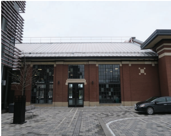
Standing seam metal roof on west elevation (ERA 2023)
