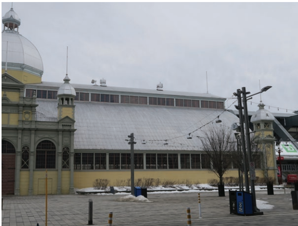
North upper roof: west section (ERA 2023)
