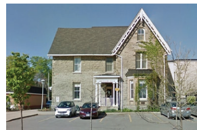
954 Bank Street (Google, 2015).
