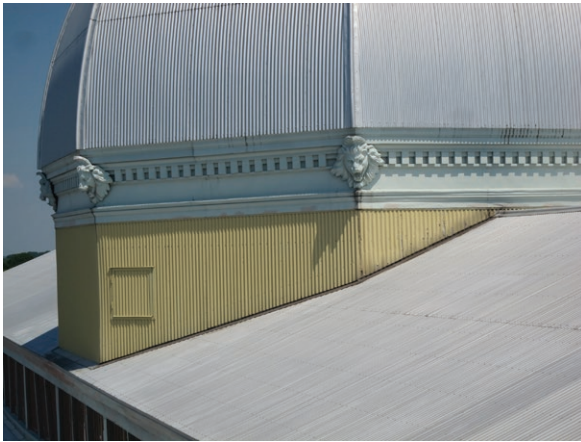
Base of roof dome from north side (ERA 2019)
