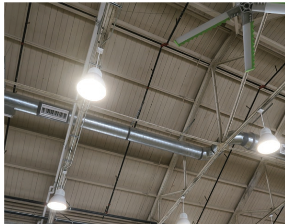
Metal truss and wood decking ceiling (ERA 2023)
