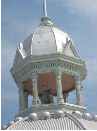
Roof cupola from south (ERA 2019)
