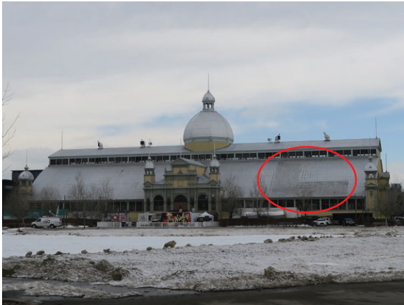
South lower roof. Note fabric covering (ERA 2023)
