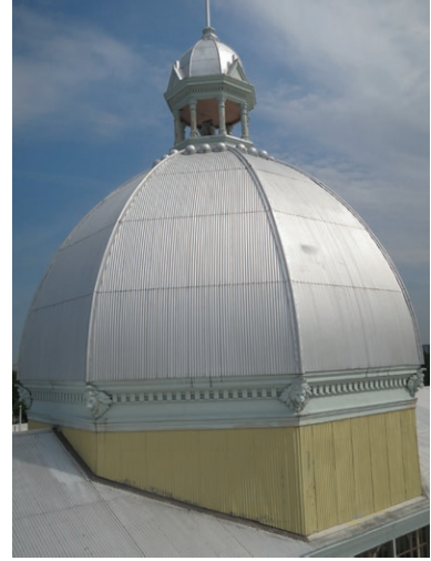
South view of roof dome (ERA 2019)
