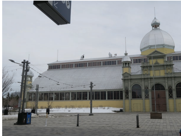
North upper roof: east section. (ERA 2023)
