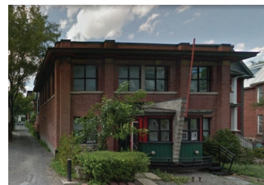
115-117 Holmwood Avenue (Google, 2016).
