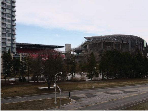
Looking southeast from the Bank Street Bridge towards TD Place (ERA, 2023).
