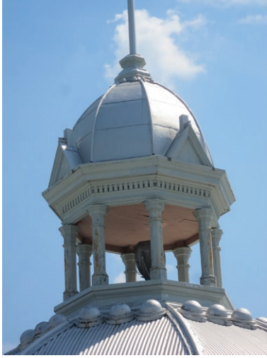
Dome roof cupola from north side (ERA 2019)
