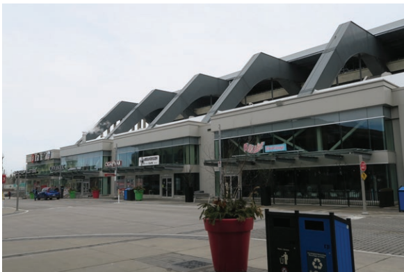
Eastern portion of the podium on the primary (north) elevation of TD Place (ERA, 2023).
