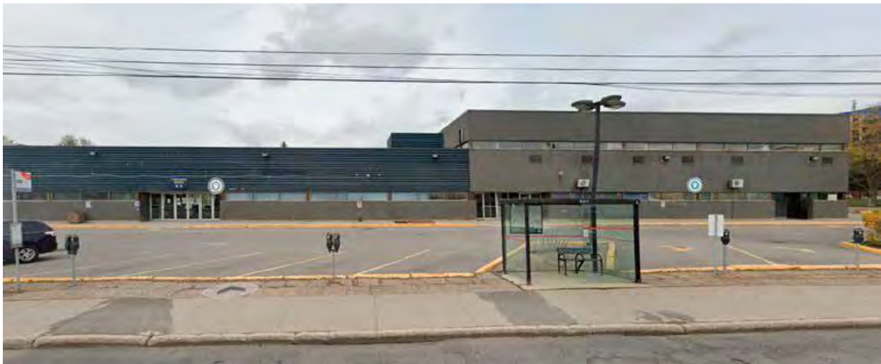
Figure 1 – Former Ottawa Bus Depot (Catherine Street Elevation)
