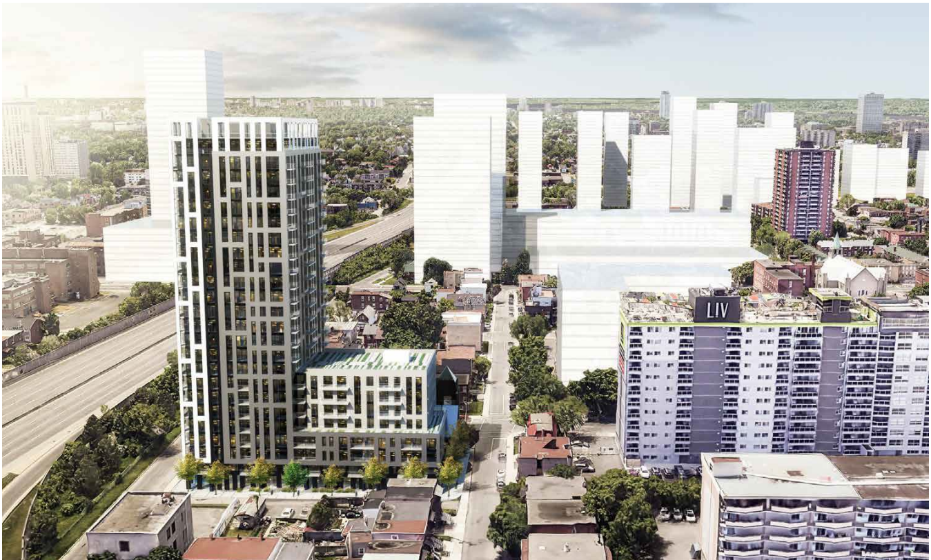
Figure 14: Context view looking northwest toward the proposed development (prepared by Neuf Architects)
