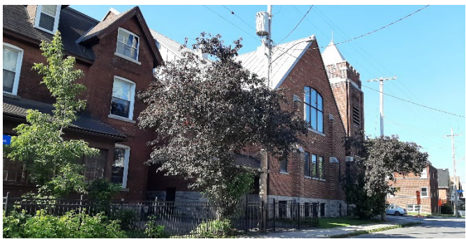
Figure 1: The walls of the north and west façade of the church, shown in the right of the photo, are proposed to be retained and the two (2) storey brick dwelling to the east of the church, shown in the left of the photo, is proposed to be demolished
