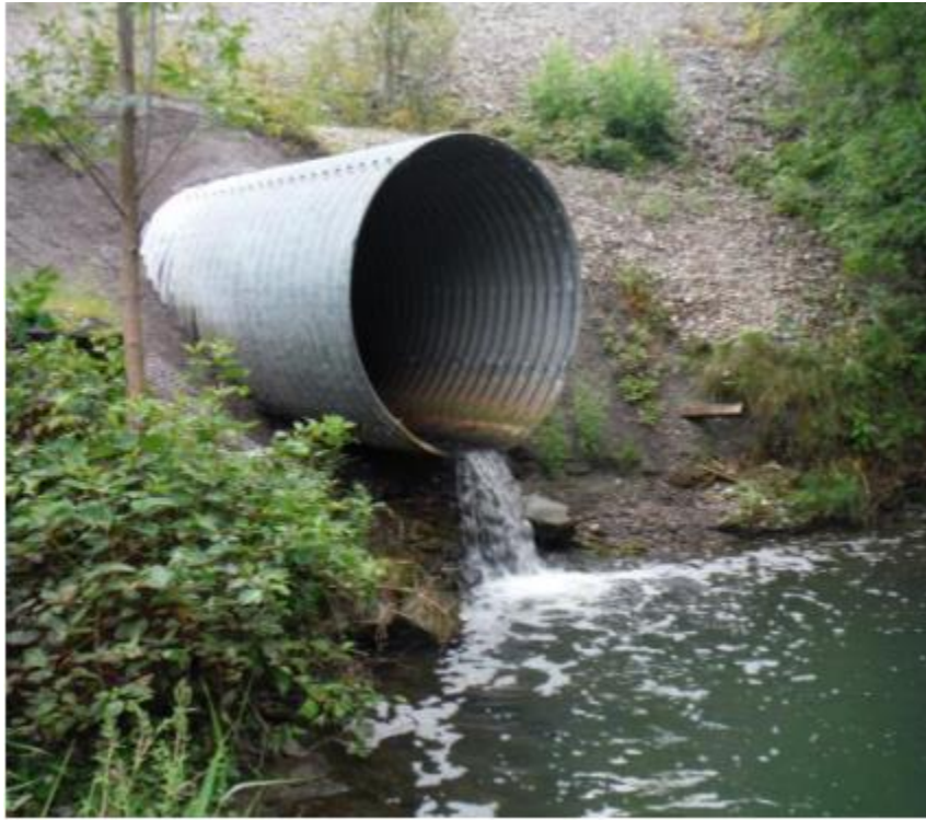
Photo 2: Perched culvert that conveys flow of Stillwater Creek under the Beachburg railway (RVCA, 2015)
