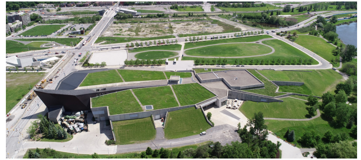
Figure 5: View of the Canadian War Museum, north of the Flats.
