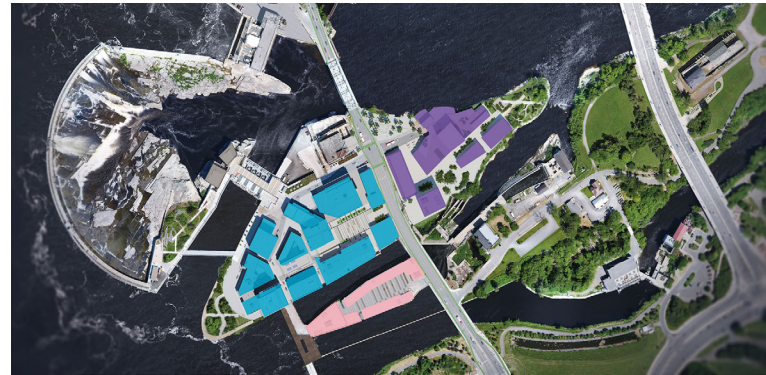
Figure 7: Chaudière and Albert Islands (Zibi).
