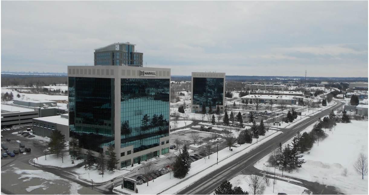
Photo 11 View of Legget Drive beyond which are surrounding office/hotel building properties to the east and southeast, facing southeast.
