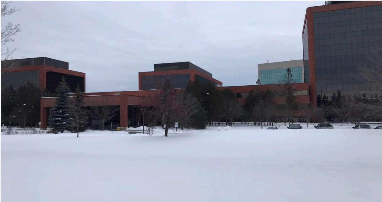
Photo 2 View of Site Buildings (Left to Right: Tower 1, Main Lobby, Tower 2, Link 2, Tower 3), facing northeast.
