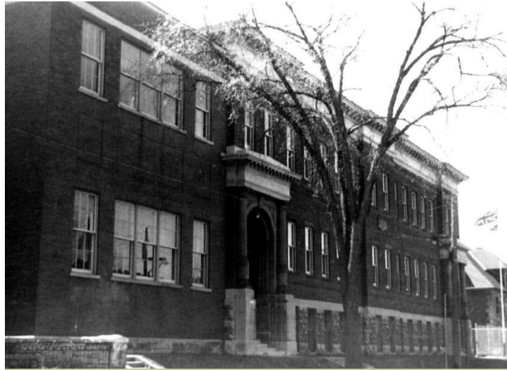
Wellington Street School, built after the fire of 1910, and located on the 665 Albert St property. Source: Ottawa Archives
