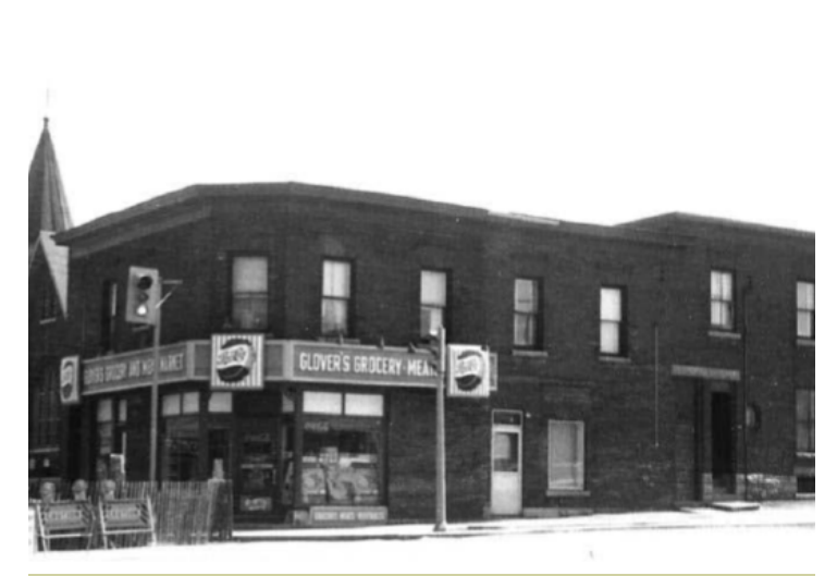
Buildings located on east side of Booth, between Albert and Wellington, 1962. Source: Ottawa Archives
