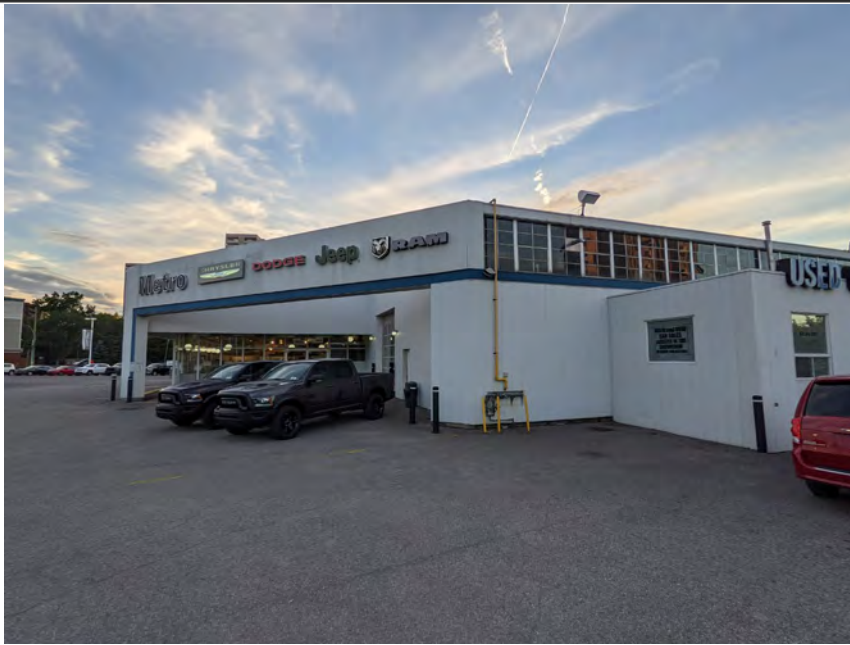
Photo 9 – Eastside of the building, facing southwest
