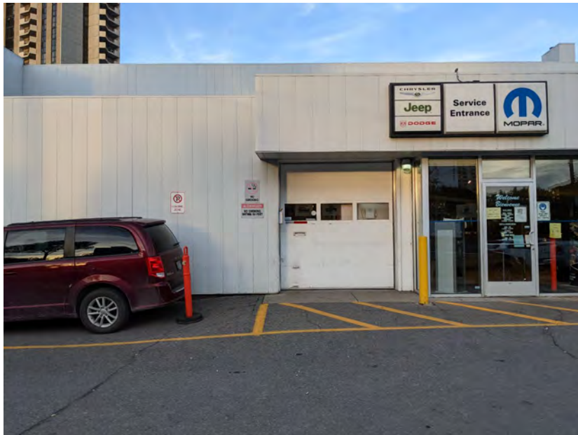
Photo 2 – Service bay entrance, westside of the building
