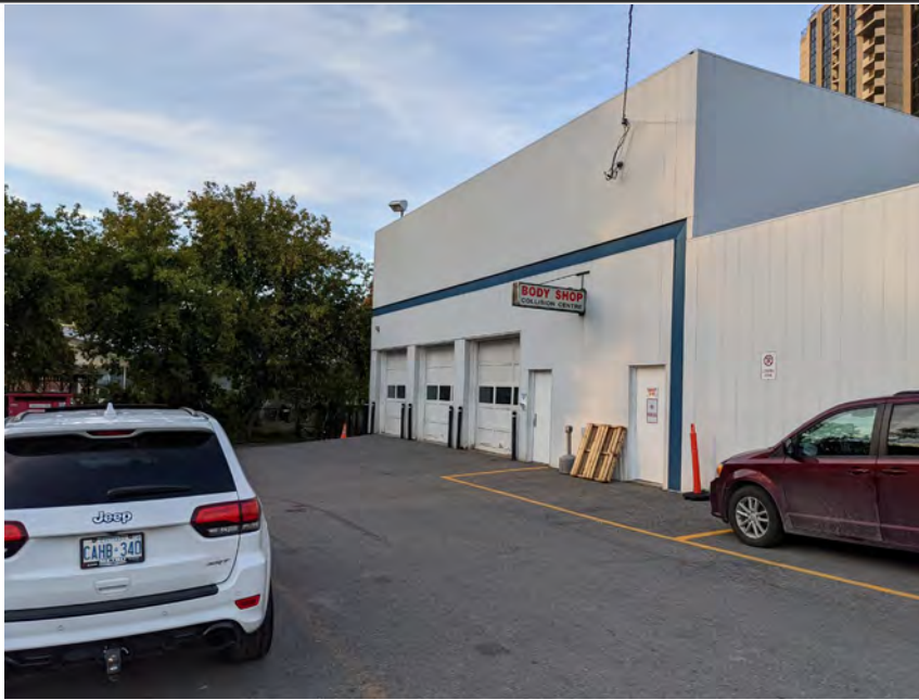
Photo 1 – Body Shop entrance, westside of the building looking north.
