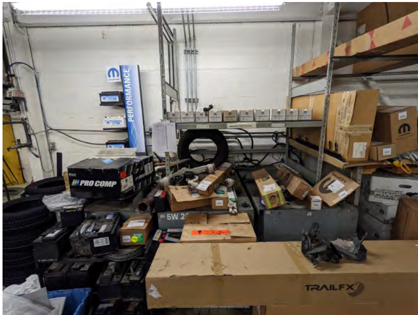
Photo 12 – Motor oil ASTs located inside the building
