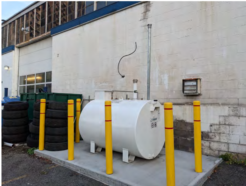
Photo 4 – Waste oil AST, north side of the building, looking southeast
