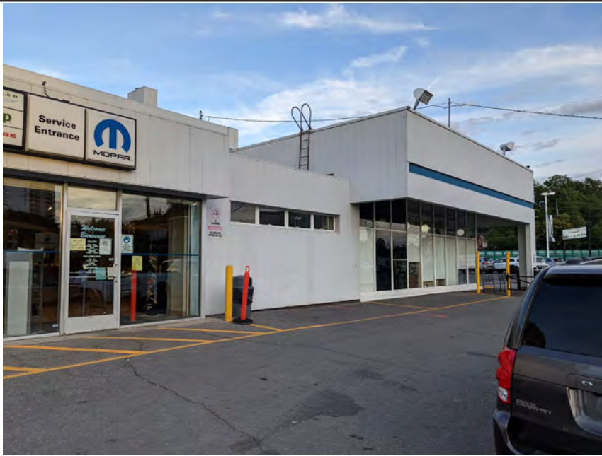
Photo 3 – West side of the building, looking north
