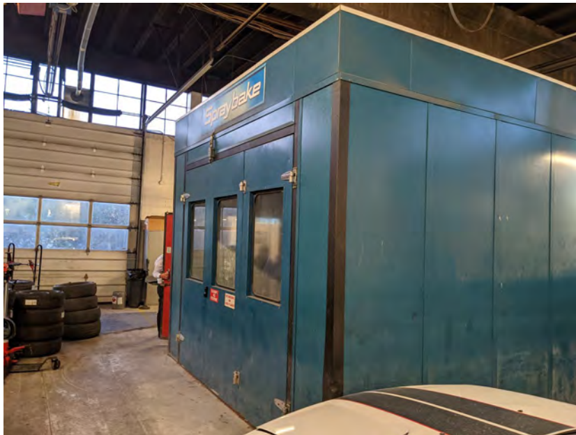
Photo 22 – Exterior of the paint booth, northside of the shop
