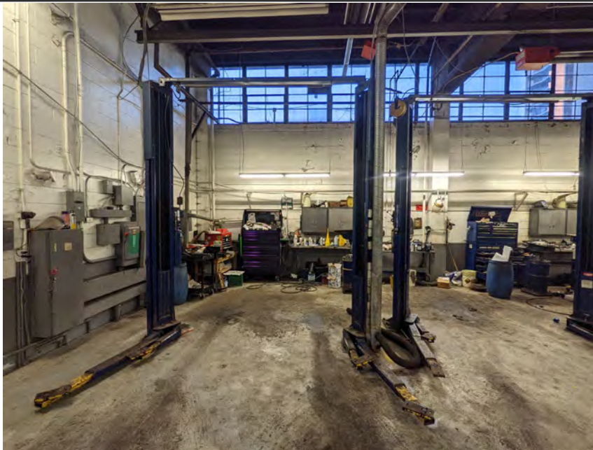
Photo 15 – Hoists in the garage, along eastside
