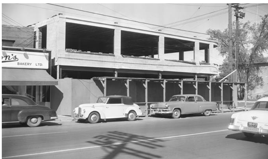
28 1191 Wellington St W, across street from site, (now World of Maps) under construction. Kitchissippi Times.
