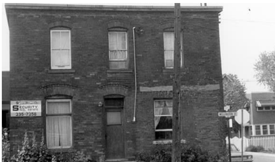
31 Photograph of residential home 963 Wellington Street West, 1968. City of Ottawa Archives, CA 26014 .
