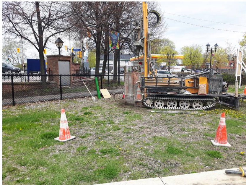
Photo 6 Looking north during drilling of MW19-01 (May 13, 2019).
