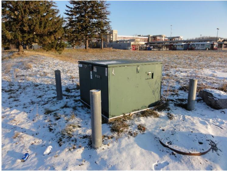
Photo 7 – View of pad-mounted transformer located on the north portion of the Site (adjacent to Woodridge Crescent).
