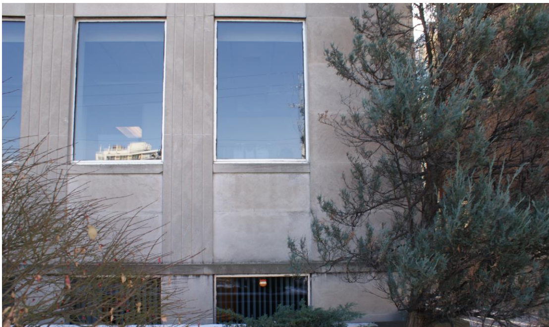
Figure 5: Detail of east elevation at the basement level. The stone belt course is cracked at the approximate mid-point of the window, and the face stone at the lower left below the window has sheared at an external corner. Source: CHRML.
