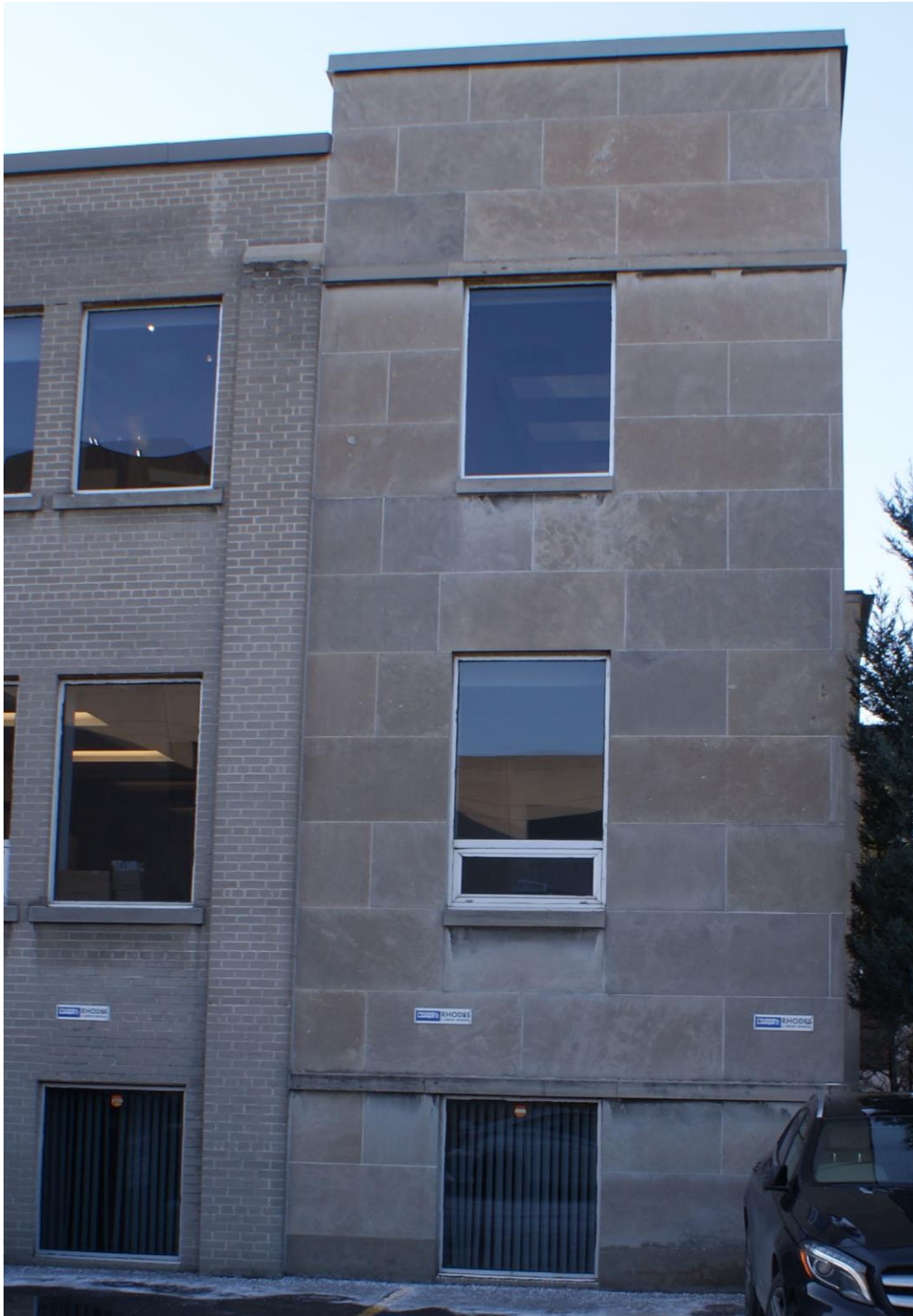
Figure 11: View of the east façade of the building. Note the lintel stone above the first floor window that overlaps onto the adjacent stones indicating a traditional load-bearing application. Note the projecting brick pilaster and its termination at the top. A steel column is likely buried behind the pilaster. The beam may support additional horizontal steel beams that would support the parapet, which the continuous shelf angle evident below the parapet belt course would be attached. Source: CHRML.
