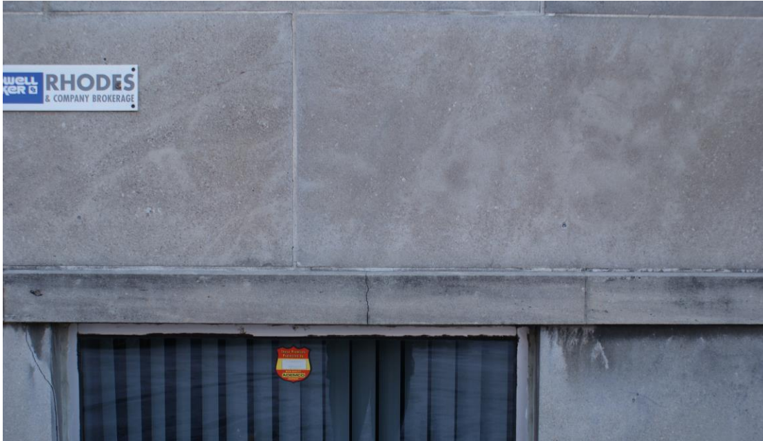
Figure 5: Detail of east elevation at the basement level. The stone belt course is cracked at the approximate mid-point of the window, and the face stone at the lower left below the window has sheared at an external corner. Source: CHRML.
