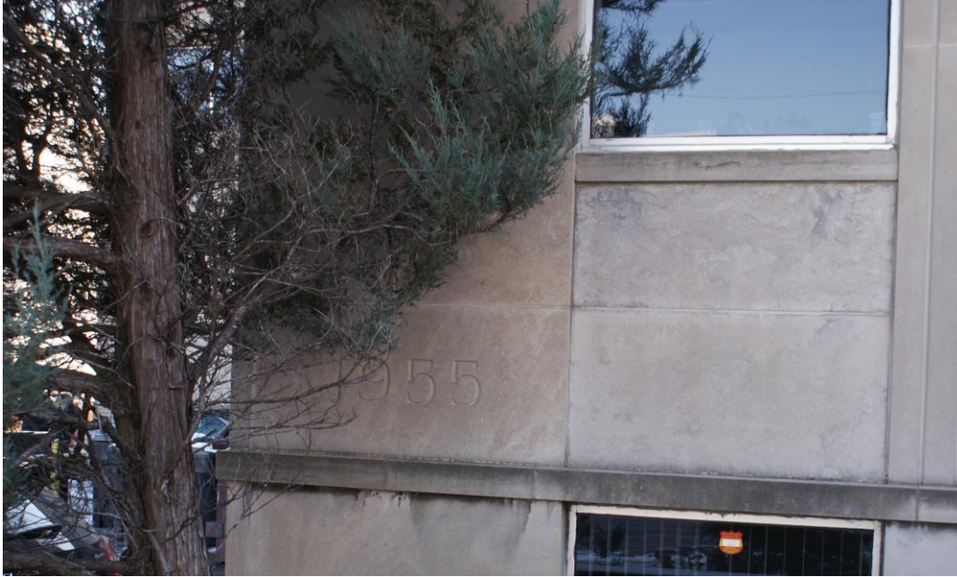
Figure 14: Detail view of stone cladding with the date stone. Note the stone sill course, windowsills, and the recessed stone panels below the windows. Source: CHRML
