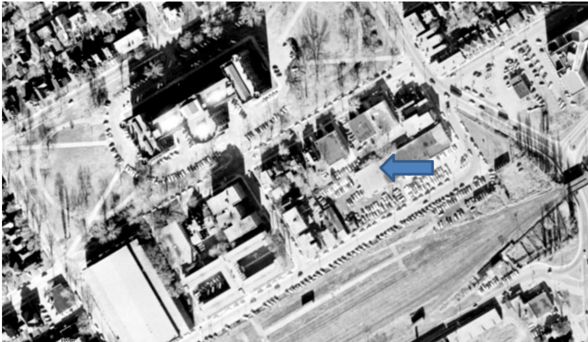
Figure 19: 1958 Aerial view of the block to the south of the Museum of Nature. The Canadian Labour Congress's new headquarters at 100 Argyle had been completed in 1955 and two other commercial buildings had been constructed to the east. Site arrowed. Source: GeoOttawa
