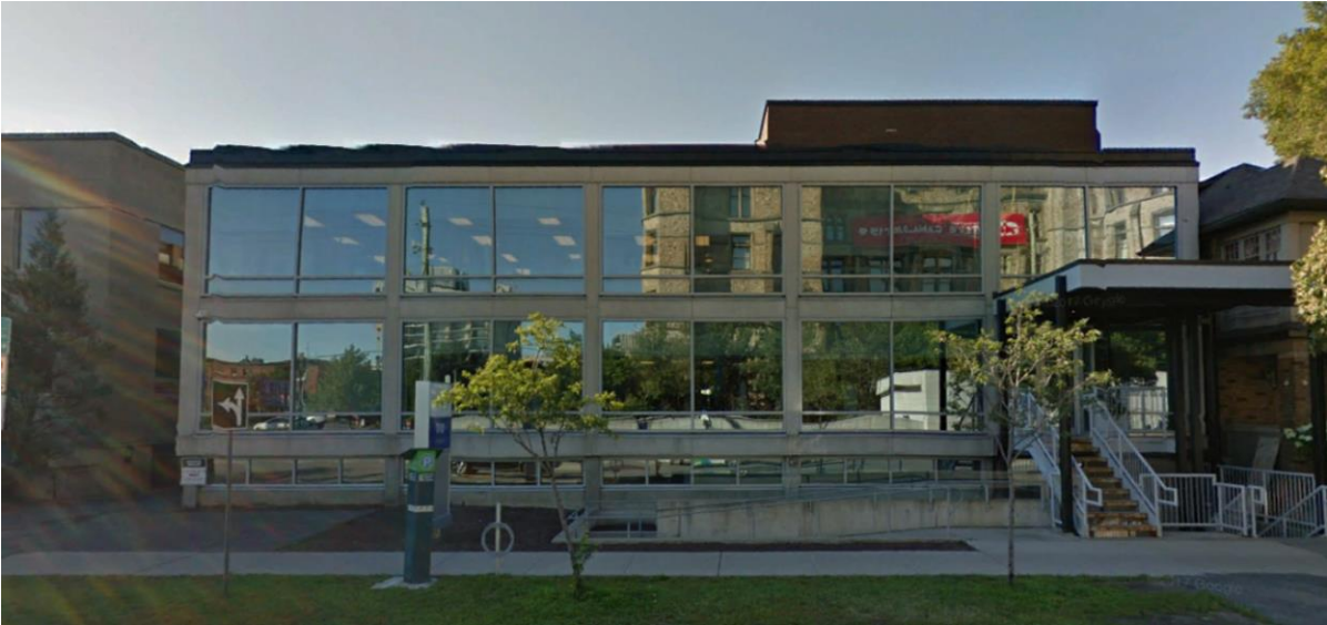
Figure 6: View of 110 Argyle the former Canadian Legion Branch 16. Source: Google Earth
