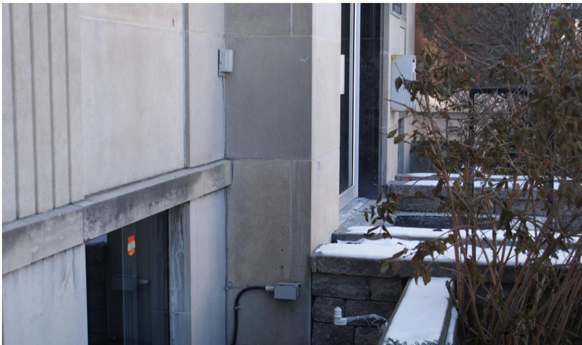
Figure 8: View of the projecting entrance bay. Note the reeded panel to the left and recessed panels below the first floor window. Source: CHRML.
