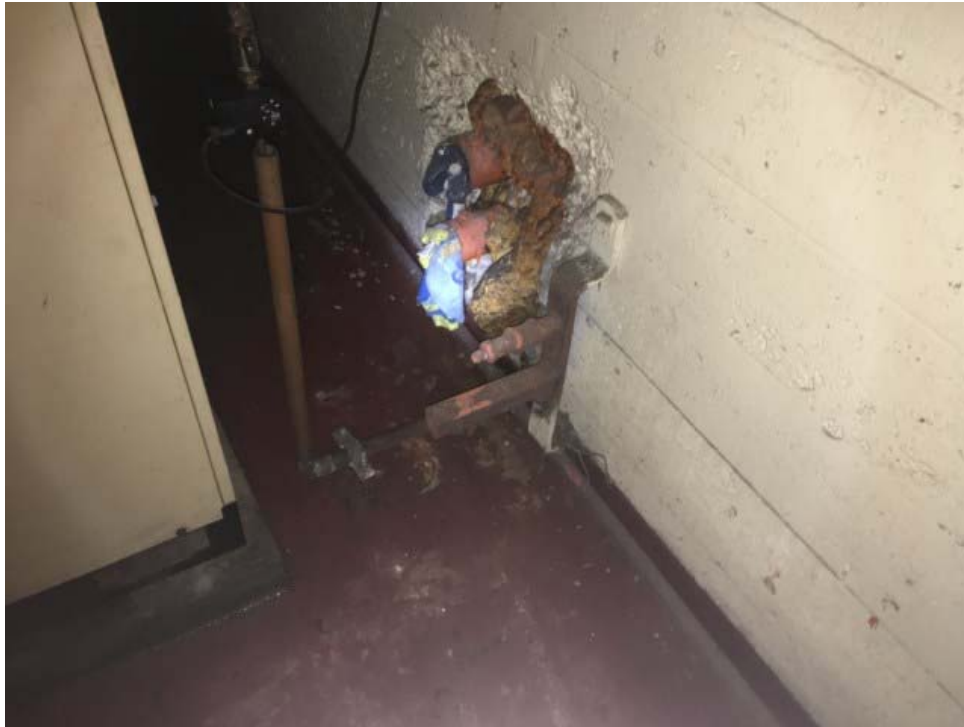
Photo 3: Two cut pipes in the eastern wall of generator room in the central heating plant this room that were likely fuel supply lines.
