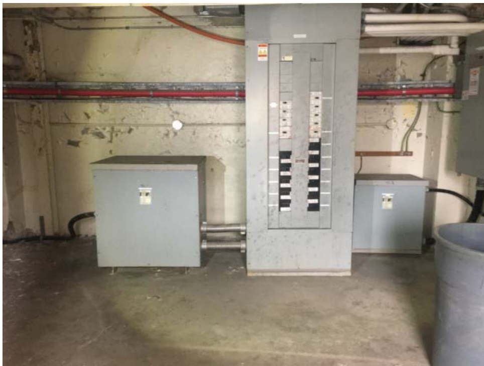
Photo 10: Typical transformers observed in the 562 Booth Street building.
