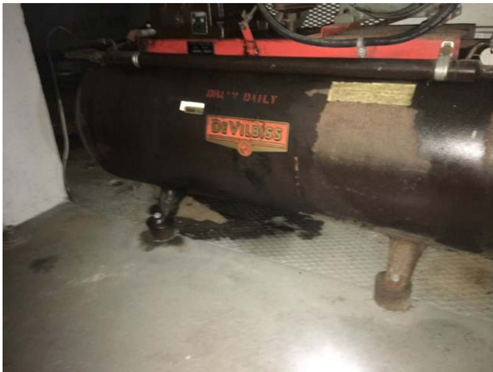
Photo 18: Leaking compressor located above a floor drain in the sub-basement level of the northern portion of the 568 Booth Street building.
