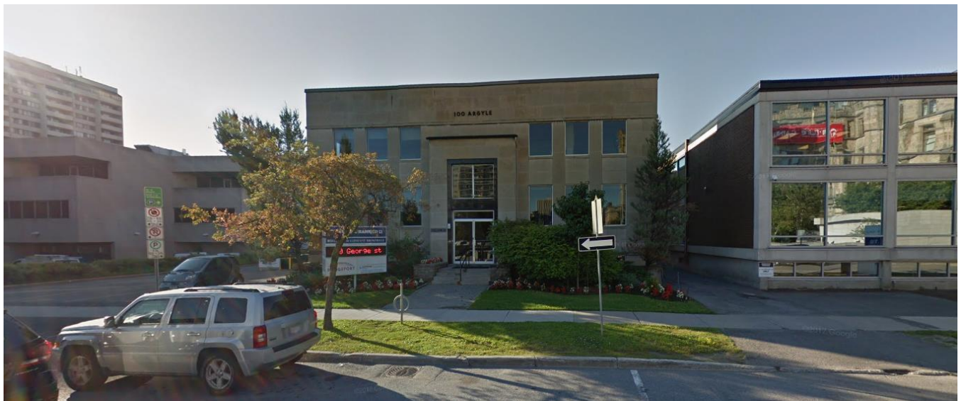
Figure 5: 100 Argyle Street, frontage and building
