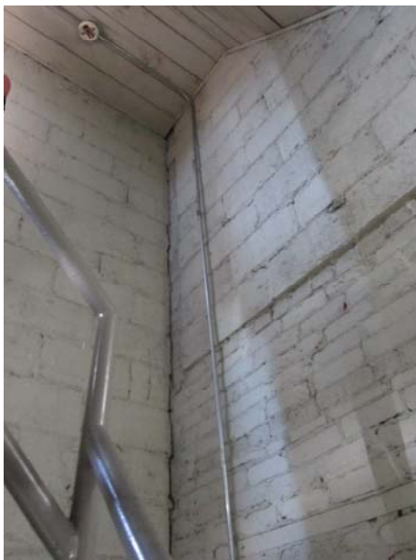
Photo 7 - Stairwell Interior at Roof
