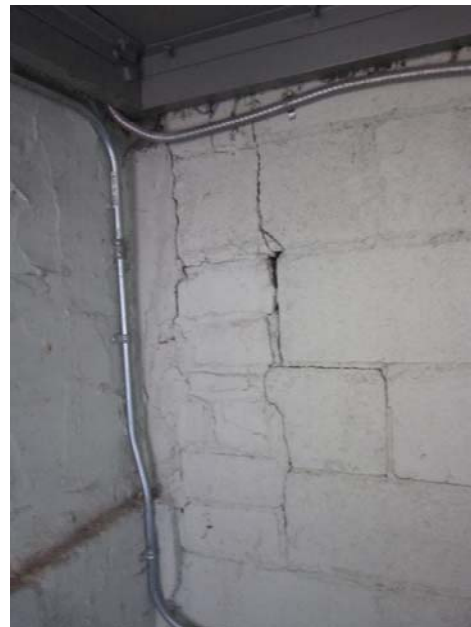
Photo 8 - Underside of Stair Landing
