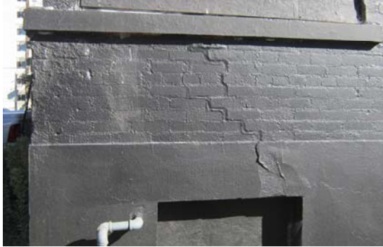
Photo 2 - South West Corner
