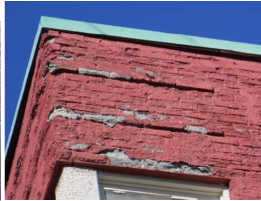
Photo 3 - South East Corner
