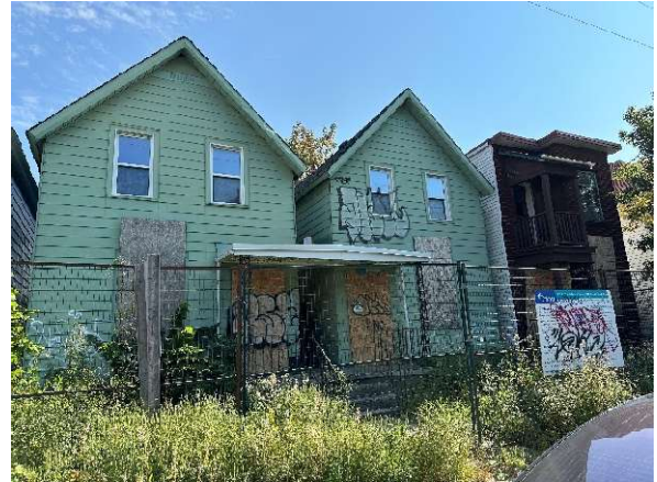
Photo 2: 277, 279 and 281 Bell St S
