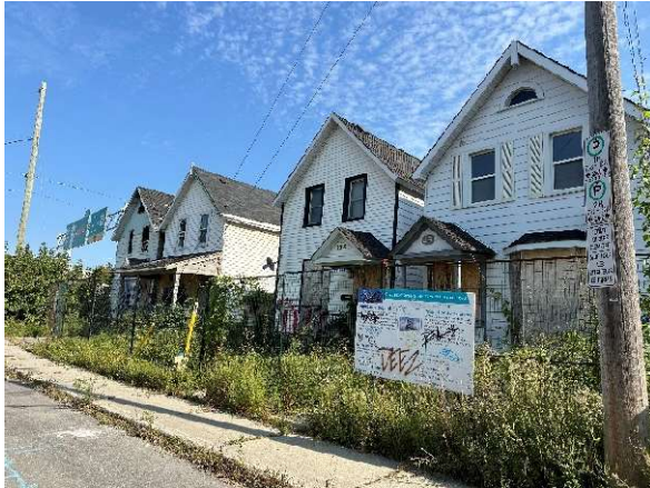
Photo 1: 269, 271, 273 and 275 Bell St S.
