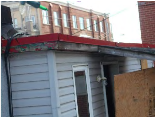
View of fascia wood rot on the two storey portion of the Site Building.
