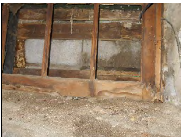
View of concrete block masonry foundation wall for the northwest portion of Site Building.
