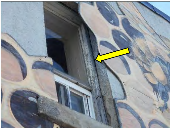
View of deteriorated window frame and sealant at perimeter of the window frame.
