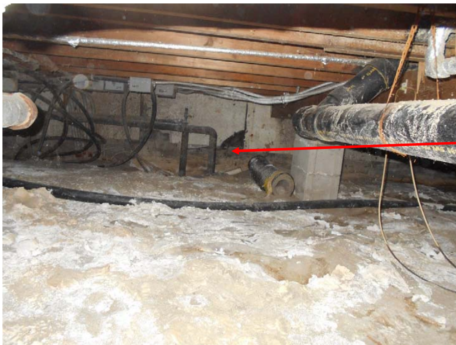
Photo 2 – North (Balsam) Building | Tar damp proofing on crawlspace walls behind Styrofoam panels
