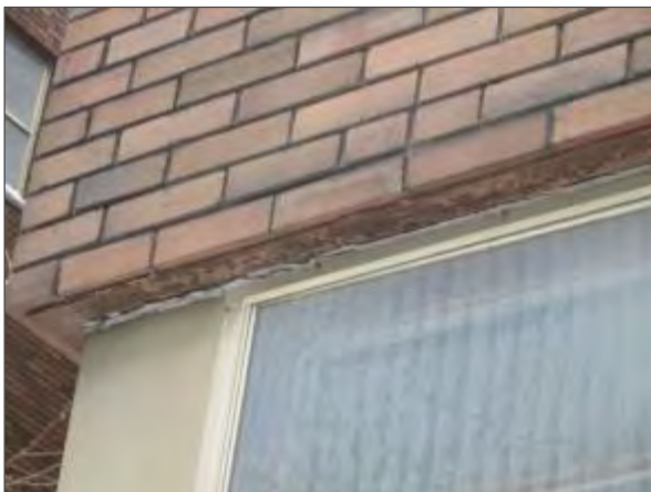
View of corrosion on a window lintel and a deteriorated perimeter window sealant observed on the south elevation of the building.
