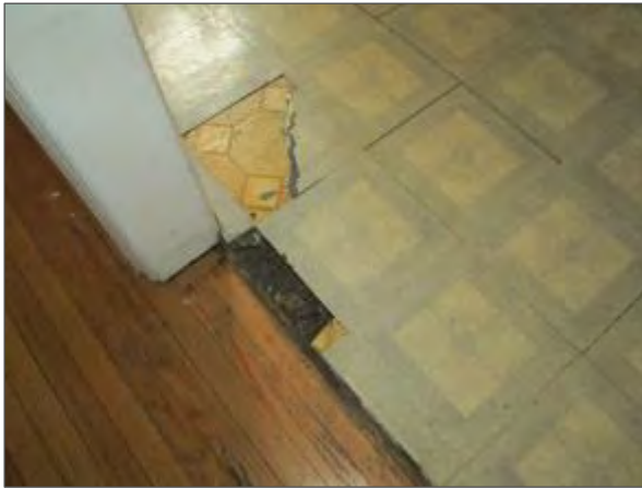
View of damaged vinyl floor tiles noted within the kitchen of suite 204.
