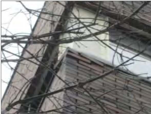
View of loose brick masonry units noted on the south elevation of the building.
