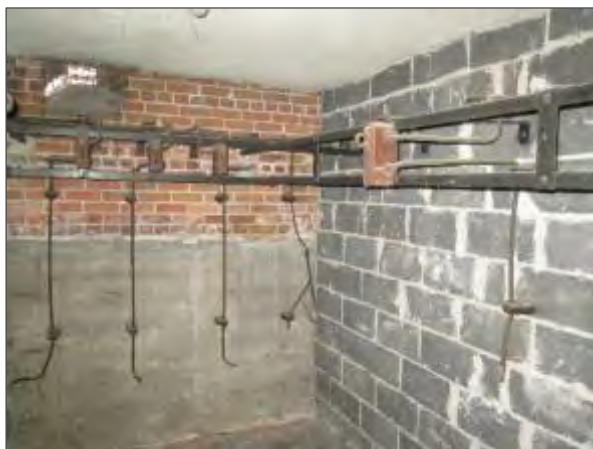
View of the abandoned knob and tube wiring system noted in the former main electrical room.
