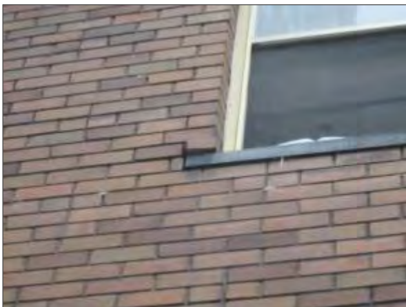
View of a loose brick masonry unit noted on the west elevation of the building.
