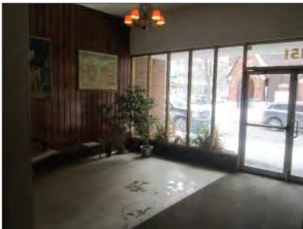
General view of the interior finishes in the main entrance lobby area.
