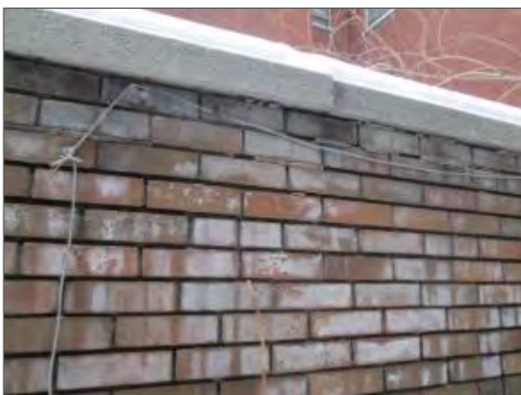
View of deteriorated mortar joints, efflorescence and a displaced concrete coping stone noted on the portion of the exterior wall which is slightly bulged.
