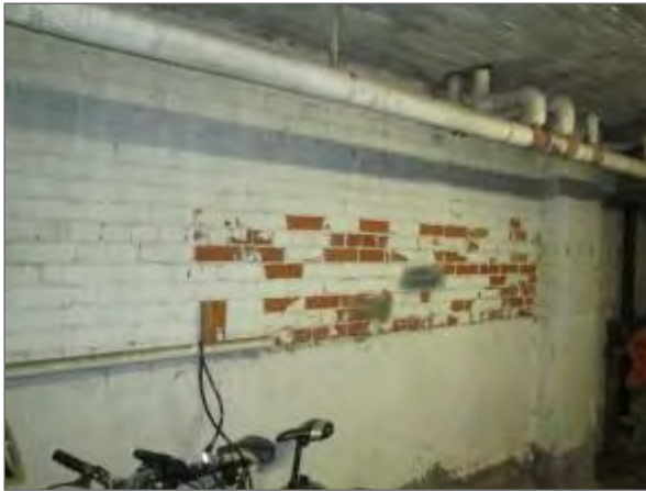
View of spalling brick masonry noted on the south foundation wall of the UPG.
