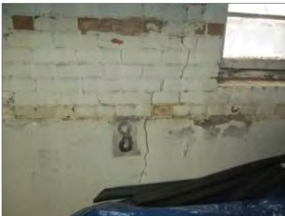
View of cracking noted in the cast-in-place concrete and brick masonry foundation walls on the south portion of the UPG.
