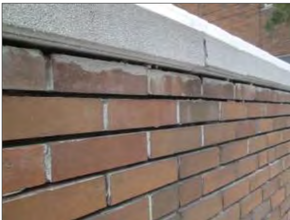
View of deteriorated mortar joints noted within the brick masonry on the south elevation of the building.
