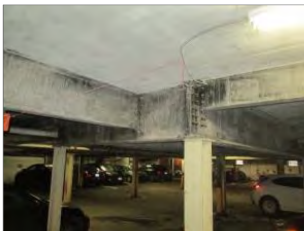
View of the steel beams and columns located in the UPG of the building which support the central portion of the building.
