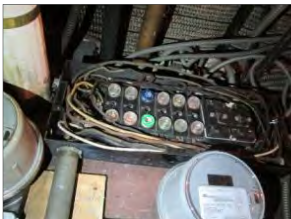
View of a glass plug fuse electrical panel noted in the main electrical room.
