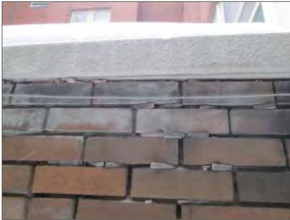
View of deteriorated mortar joints noted in the brick masonry on the south elevation and a crack in the concrete coping stone.
