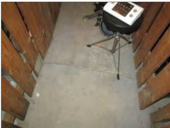
View of cracking noted in the concrete floor slab in a basement locker room.
