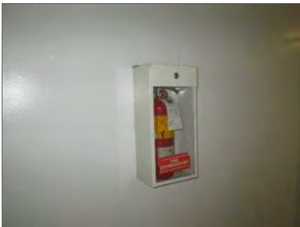
View of the typical cabinet mounted chemical fire extinguishers serving the Site Building.
