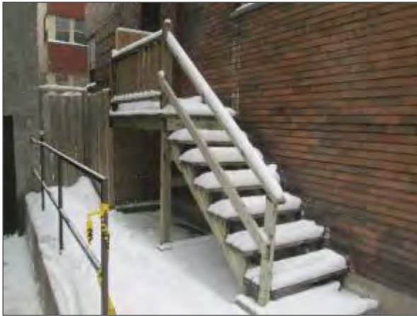
View of the wood framed staircase located on the north elevation of the building.
