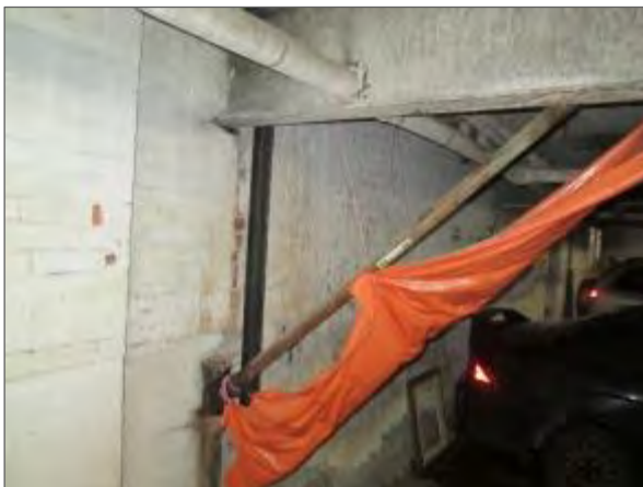
View of an orange tarp which is being used to divert leaking water from the UPG roof deck to the perimeter of the UPG.
