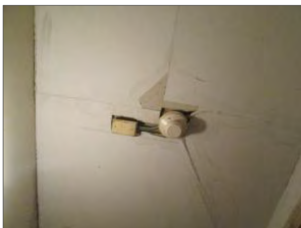
View of damaged gypsum ceiling finishes noted near the roof access door.
