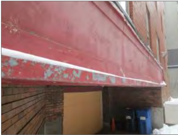
View of deteriorated paint finishes noted on the metal cladding above the overhead door serving the UPG on the east elevation of the building.
