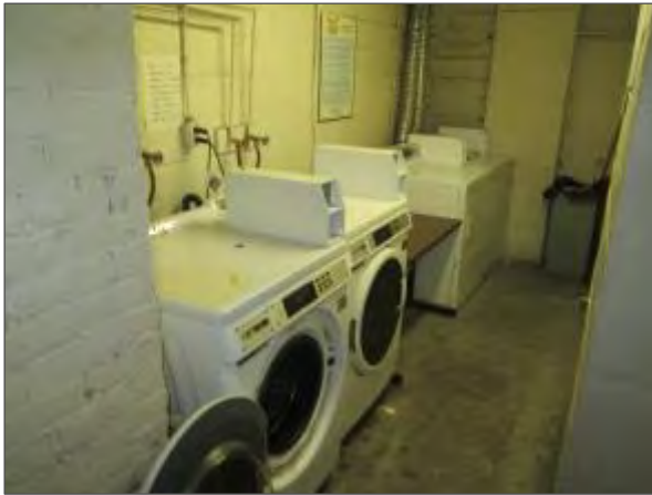
General view of the basement level laundry room.
