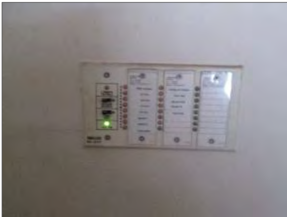
View of the annunciator panel which is located in the main entrance lobby area.
