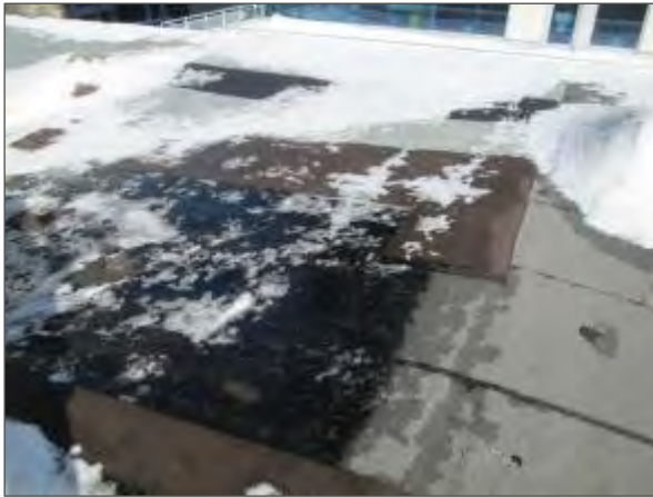
View of several patch repairs noted on the main roof of the building atop the fourth floor.
