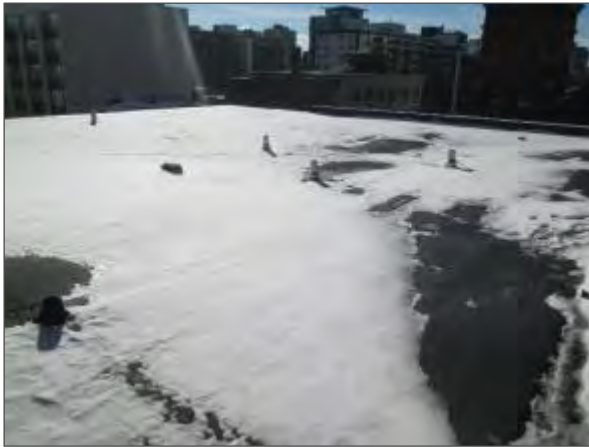
View of a portion of the main roof system atop the fourth floor of the building.
