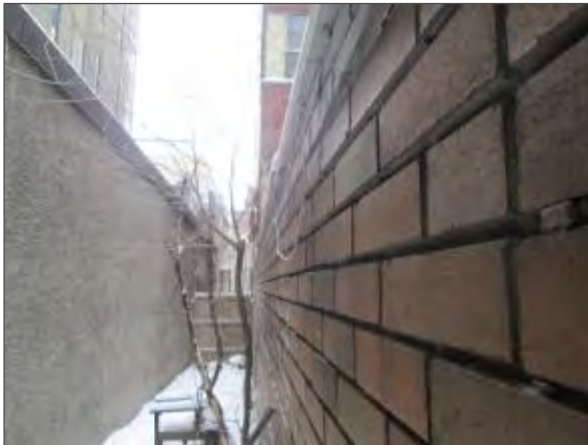
View of an area of brick masonry on the north elevation of the building (wall which flanks the UPG) which has a slight bulge.
