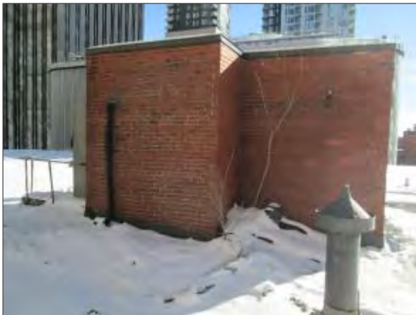
View of vegetative growth noted near the exterior wall of the stairwell penthouse on the main roof.
