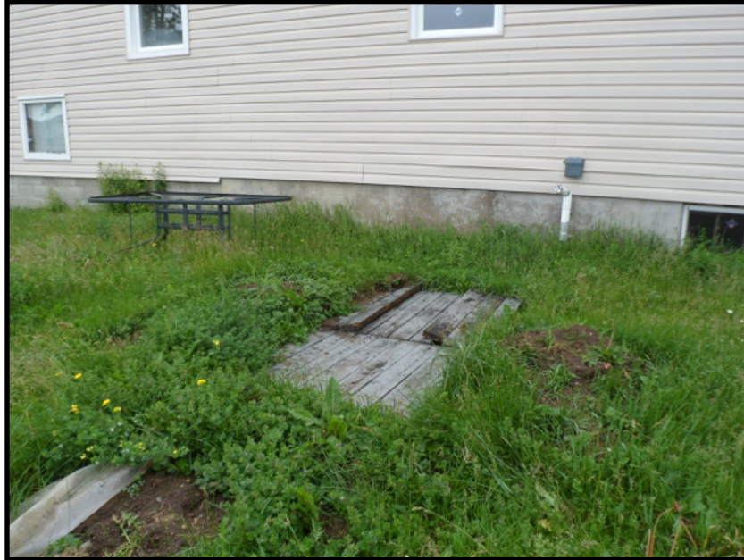
Photo 3: Showing the septic area located on the west side of the house on property #27.
