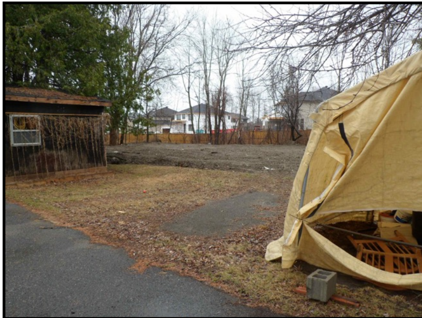
Photo 22: View to the west of the outbuildings located at property #35 Scissons Road
