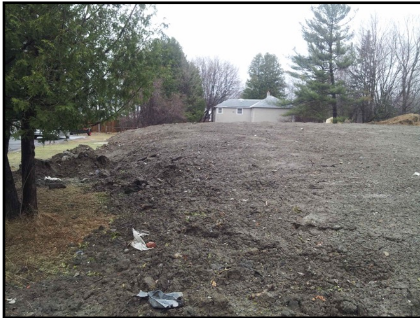
Photo 13: View to northwest across property #33 Scissons Road showing the copse of cedars and the original ground surface on the left side of the photo and the fill over the rest of the property.
